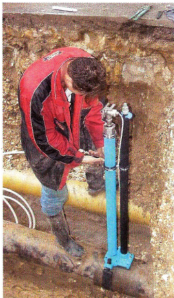
Figure 4: Sensor installed with special Schacht module
