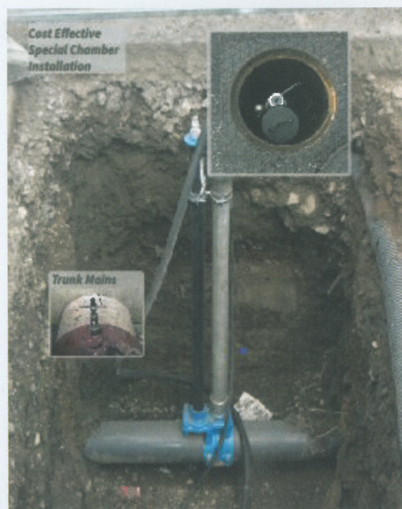
Figure 5: Sensor installed with special Schacht module
